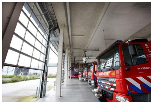
Fire station Enschede - Netherlands
